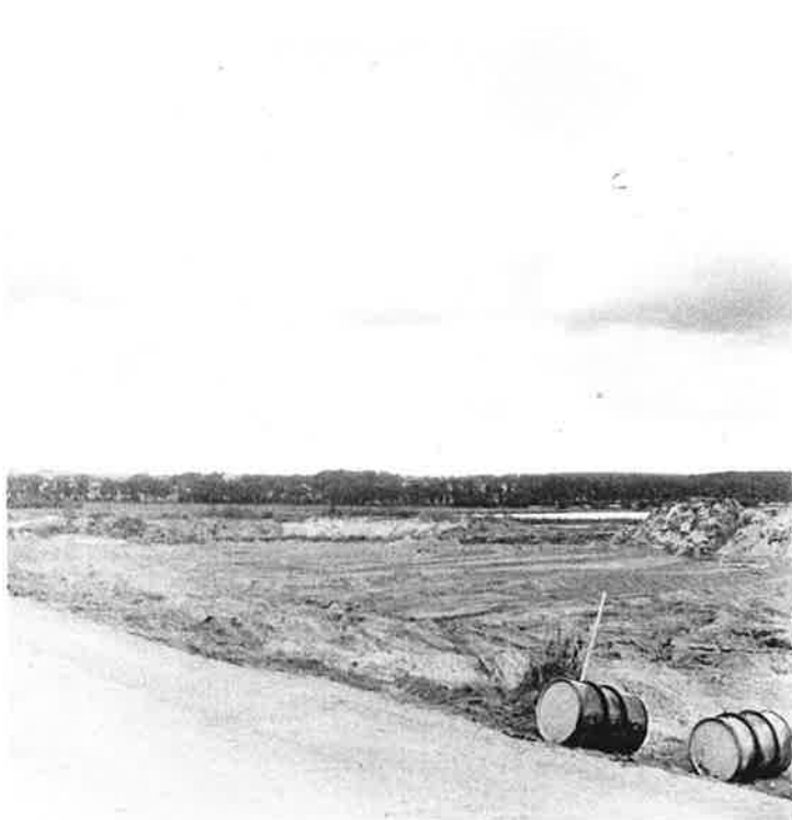
Fig. 28. View of the station from the road on August 15, 1957.
