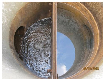
P-pond 5 : inlet (left) and outlet (right)
